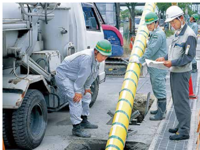
Replace aging gas pipes with polyethylene pipes
