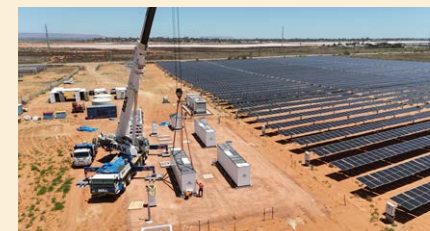
YES Group solar power plant and battery storage facility currently under construction
