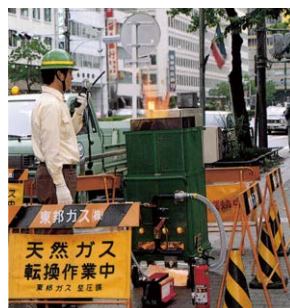
LNG conversion work near Nagoya Station
