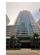
TOHO GAS SINGAPORE office building
