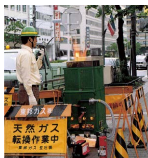
LNG conversion work near Nagoya Station
