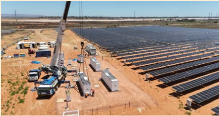
YES Group solar power plant and battery storage facility currently under construction
