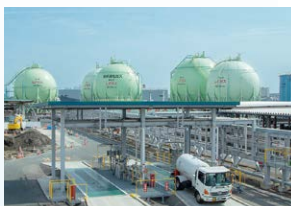
Toho Liquefied Gas Co., Ltd., Meiko LPG Terminal
