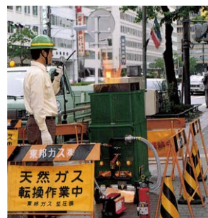
LNG conversion work near Nagoya Station
