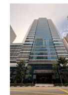
TOHO GAS SINGAPORE office building
