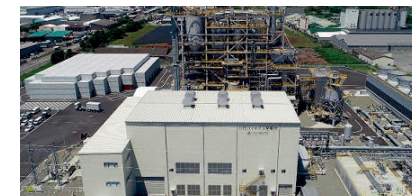
Yatsushiro Biomass Power Plant (Operations commenced in June 2024)
