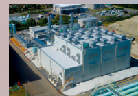
Yokkaichi Power Plant
