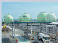
Toho Liquefied Gas Co., Ltd., Meiko LPG Terminal
