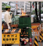
LNG conversion work near Nagoya Station
