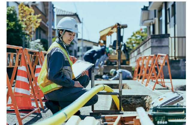
Trenchless pipe installation method
