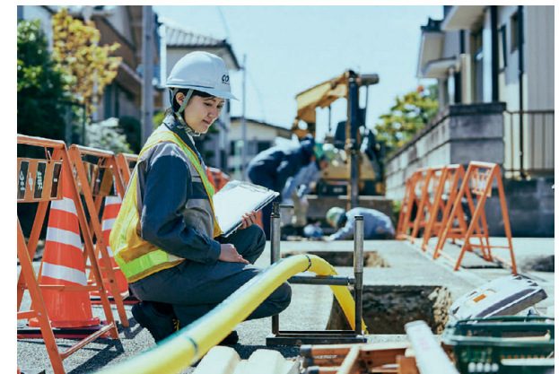
Trenchless pipe installation method
