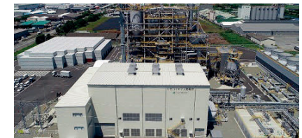
Yatsushiro Biomass Power Plant (Operations commenced in June 2024)
