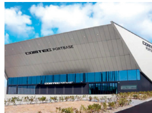
COMTEC PORTBASE (opened earlier in the Phase II area of Minato AQULS)
