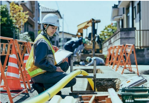
Trenchless pipe installation method
