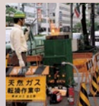
LNG conversion work near Nagoya Station
