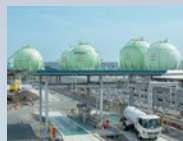
Toho Liquefied Gas Co., Ltd., Meiko LPG Terminal
