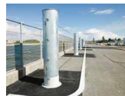
The tsunami screen protects plants from flying flotsam
