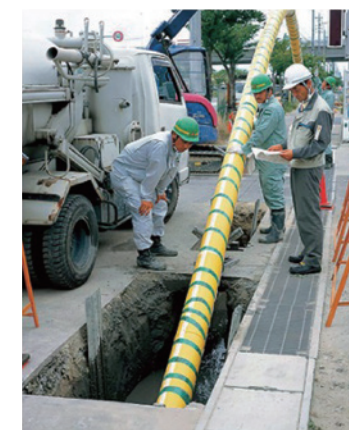
Trenchless pipe installation method
