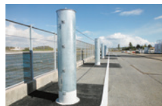
"Tsunami screen" as a countermeasures against flotsam from factories
