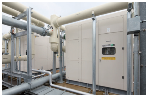
Two highly efficient, natural chiller units
