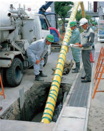
Trenchless pipe installation method
