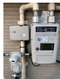
Remote meter-reading device
