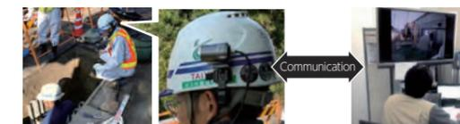
Remote site verification using a wearable camera
