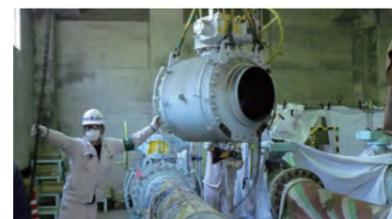
Measures against aging at gas manufacturing works (valve replacement on a main gas transmission pipeline)
