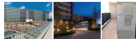
Park Homes LaLa Nagoya Minato AQULS (left and center: exterior, right: Enefarm)
