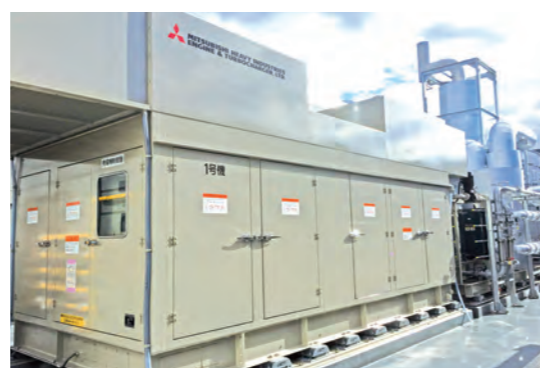
Gas cogeneration system with a BOS* function *Blackout start: A function to start up engine and supply electricity without using an external power supply source
