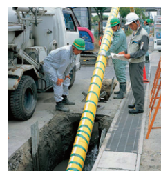
Trenchless pipe installation method
