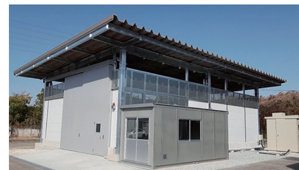
Hydrogen combustion test conducted at Technical Research Institute
