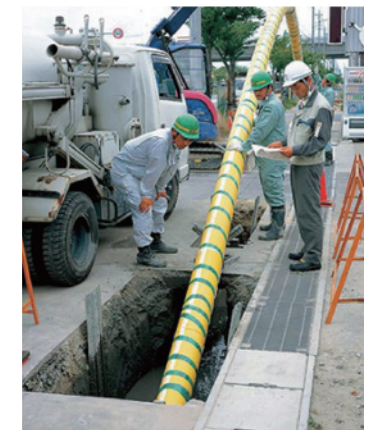
Trenchless pipe installation method
