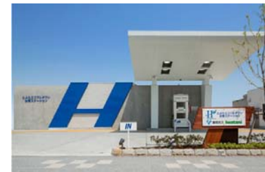
[Hydrogen refueling station]
