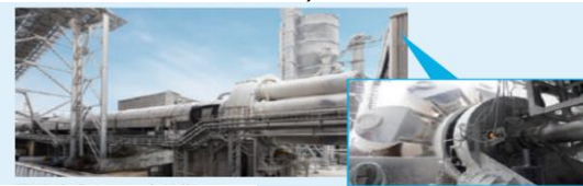
Overall view of lime combustion kiln
