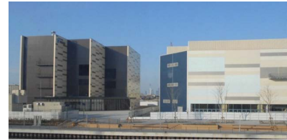
Energy center (left) and Shopping mall LaLaport (right) (located in “Minato AQUUS”)
