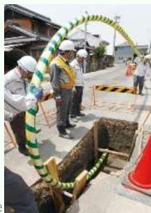
Adoption of earthquake-resistant pipes
