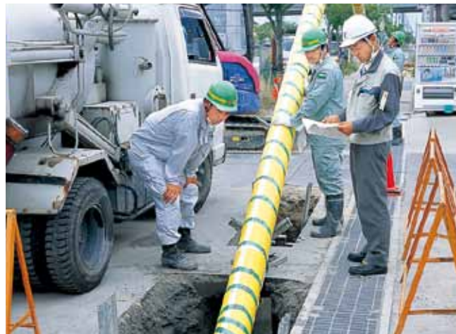
Replace aging gas pipes with polyethylene pipes
