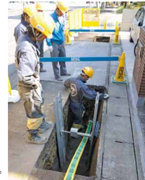
To reduce the amount of dirt unearthed during the installation of pipelines, Toho Gas uses a trenchless method that rips up only small parts of the road surface.
