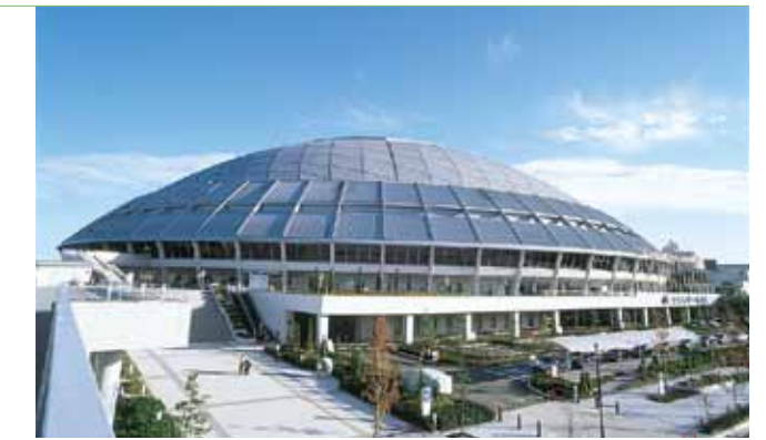
Nagoya Dome which introduces gas-absorption water chillers/heaters
