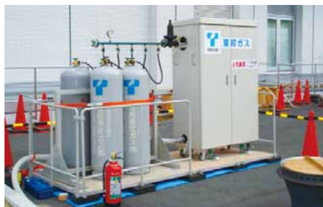
Movable gas generating facilities
