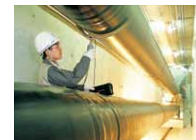
Transport trunk line installed in public utility conduit
