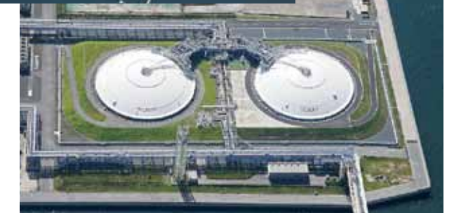
One of the world's largest in-ground tanks with a capacity of 200,000 kiloliters is located at the Chita-Midorihamma Works. The amount stored here is equivalent to the annual consumption of 300,000 average households.
