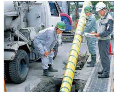
Replace aging gas pipes with polyethylene pipes
