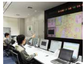
Automatic supply management system
