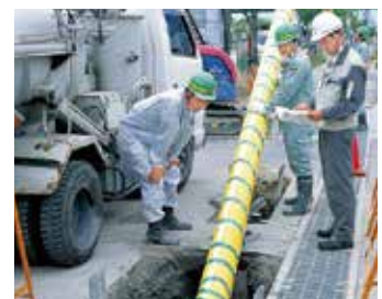
Replace aging gas pipes with polyethylene pipes
