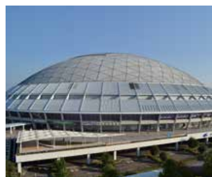
Air Conditioning System for Commercial Use
