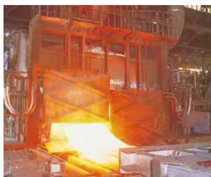
Industrial Furnace for Industrial Use
