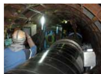
Constructing the "Cross Ise Bay Gas Pipeline"
