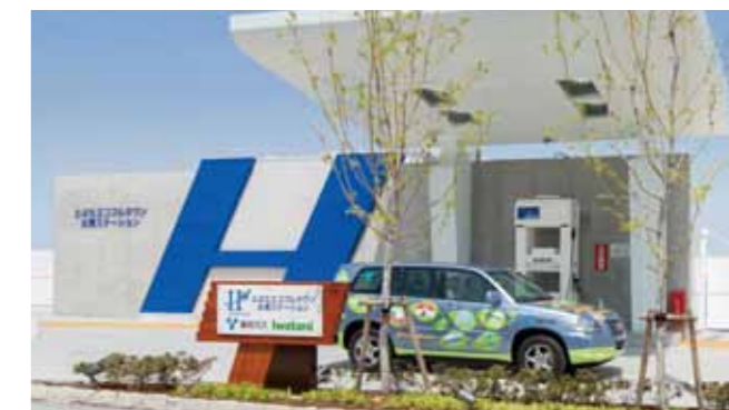
Hydrogen refueling station
