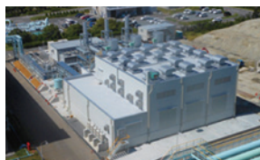
Yokkaichi Power Station
