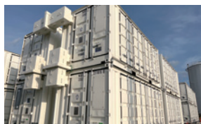
Tsu Power Station (under construction)
