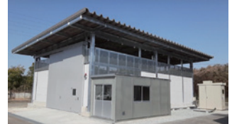
Hydrogen combustion test field at the Toho Gas Technical Research Institute
