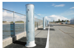
"Tsunami screen" as a countermeasures against flotsam from factories
