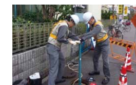
Low-pressure gas shutoff system installation work
