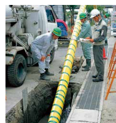
Trenchless pipe installation method
