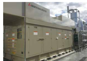
Gas cogeneration system with a BOS* function
