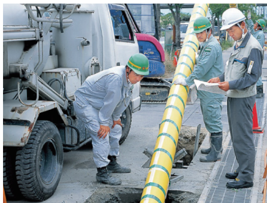
Replace aging gas pipes with polyethylene pipes
