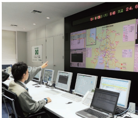
Automatic supply management system
