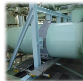
Disaster countermeasures at city gas works (reinforce LNG receiving piping)
